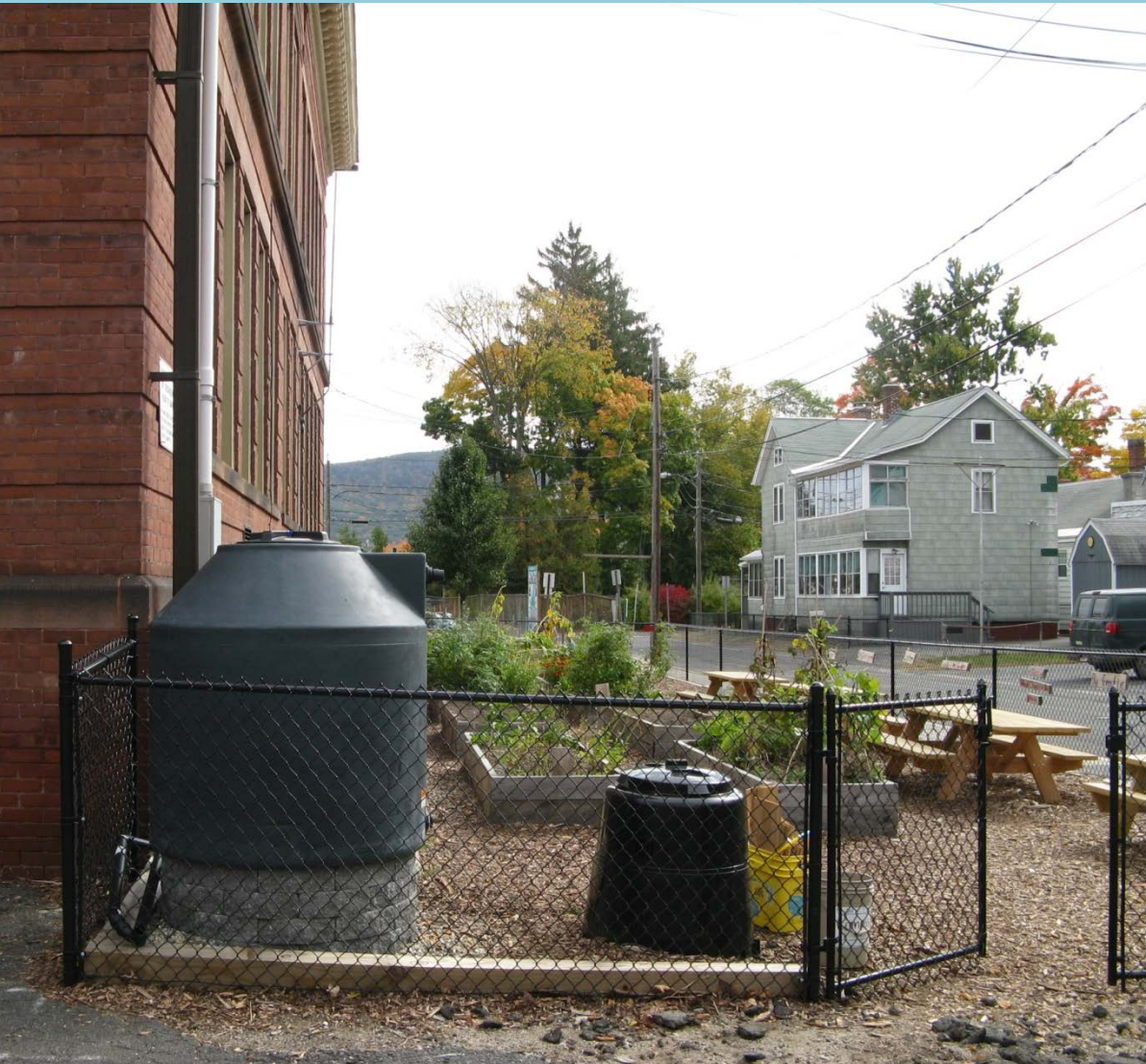
Rain water cistern, Center-Pepin School, Easthampton
